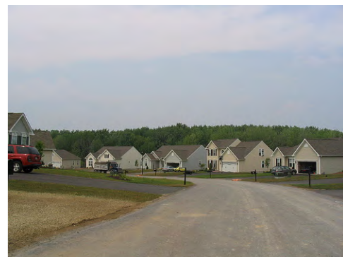
New residential construction at Sun Meadows.
