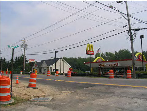
Downer Street at Crego Road.
